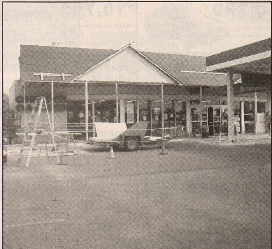
Pictured: H Squared's recent renovation to convenience store in Uvalde
