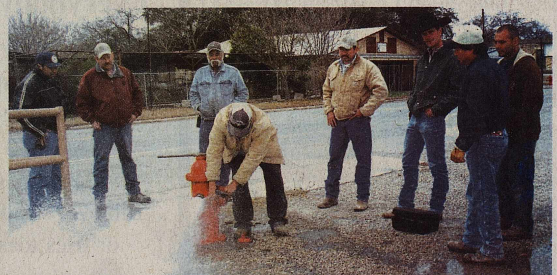
Brackett News Photo By Leigh Volcsko - City of Brackettville Maintenance Employee Javier DeLeon tests the water pressure of a city hydrant during a maintenance class led by A.J. Olson of Liquid Learning. Pictured from left: Marco Rodriguez (City), Refugio Martinez (FCS), Joe Kelley (City), Javier DeLeon (City), Baldamar Martinez (FCS), A.J. Olson, George Maldonado (City of LaPryor) and Abel Longoria (LaPryor).
