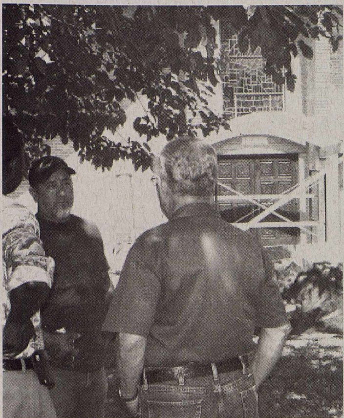
Brackett News Photo By Leigh Jenkins Volcsko - From left; Father Pius Ezeigbo, Contractor Juan Garcia and Henry Fuentes discuss the construction of the new awning recently added to St. Mary Magdalene Catholic Church. Father Pius and Fuentes shared the church had recently made improvements to parsonage, constructed a new church office, added restrooms in the sanctuary and in the future plan to update the church sign.
