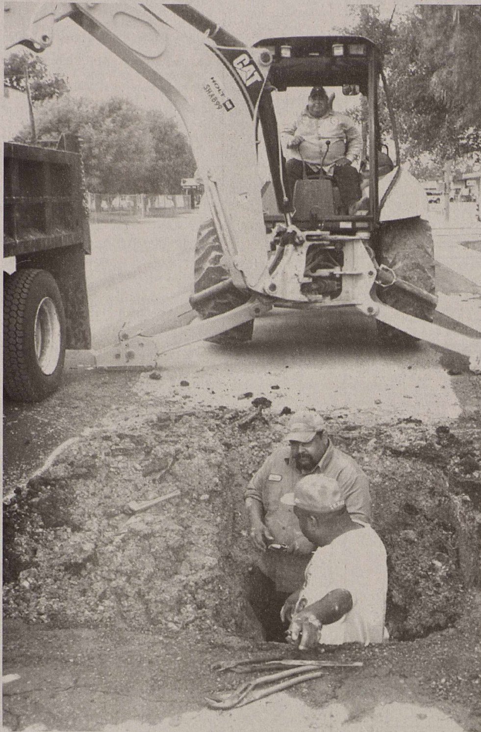
Brackett News Weekly Photo By Leigh Jenkins - City of Brackettville water works employees work to repair a leak on July 20, on Ann Street in front of the First Baptist Church.
