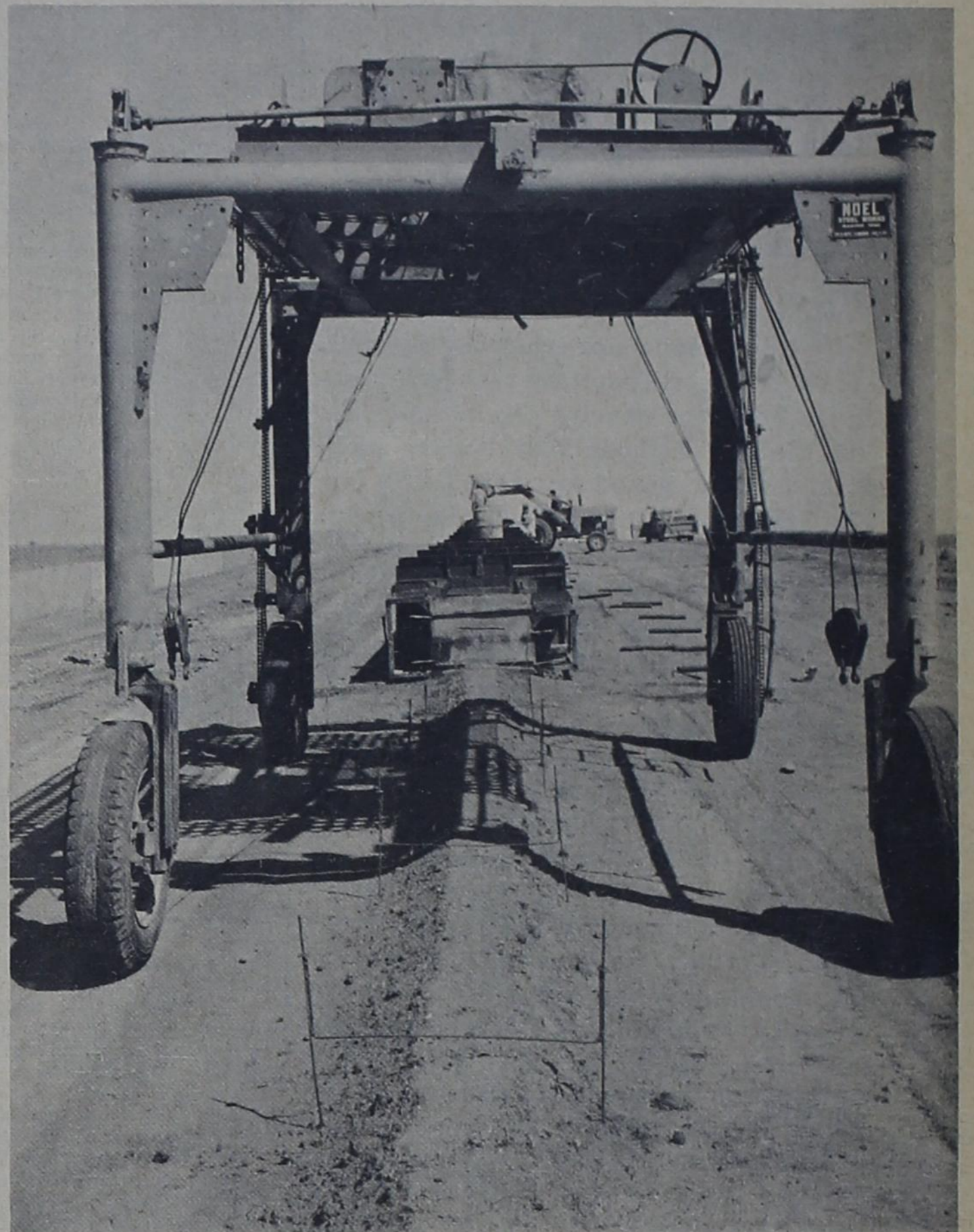
EXPANSION -- Construction is underway at Parmer County Cattle Company, southwest of Bovina, on feeding troughs for an additional 16,000 to 17,000 head of cattle. Pens will also be added at the expansion site across Running Water Draw from the present pens, mill, and offices, giving a total capacity of over 35,000 head.
