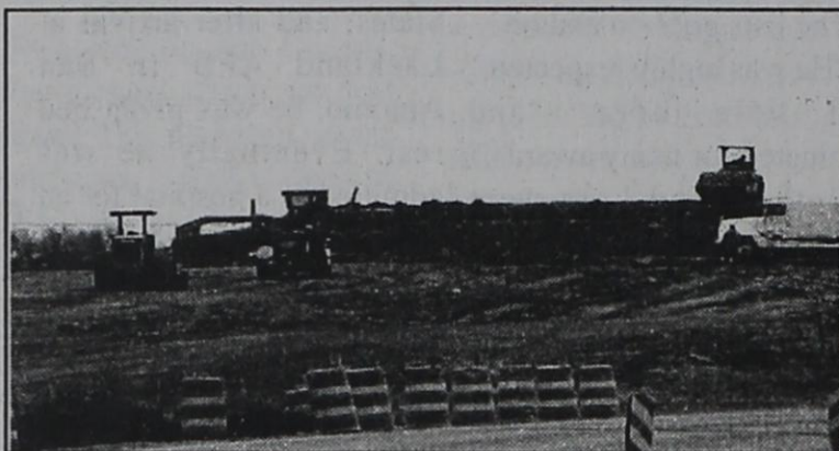
Hwy 283 Construction in Baird on the Cross Plains Hwy.
