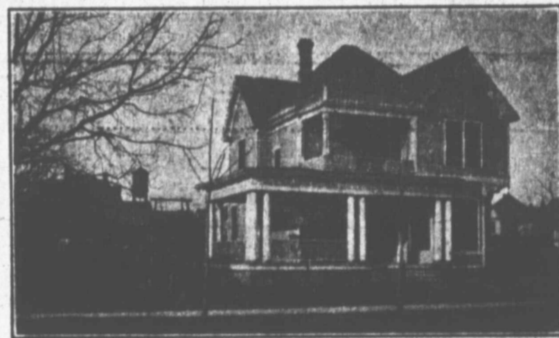
RESIDENCE OF ED. HOWARS, LAMAR AVENUE.
