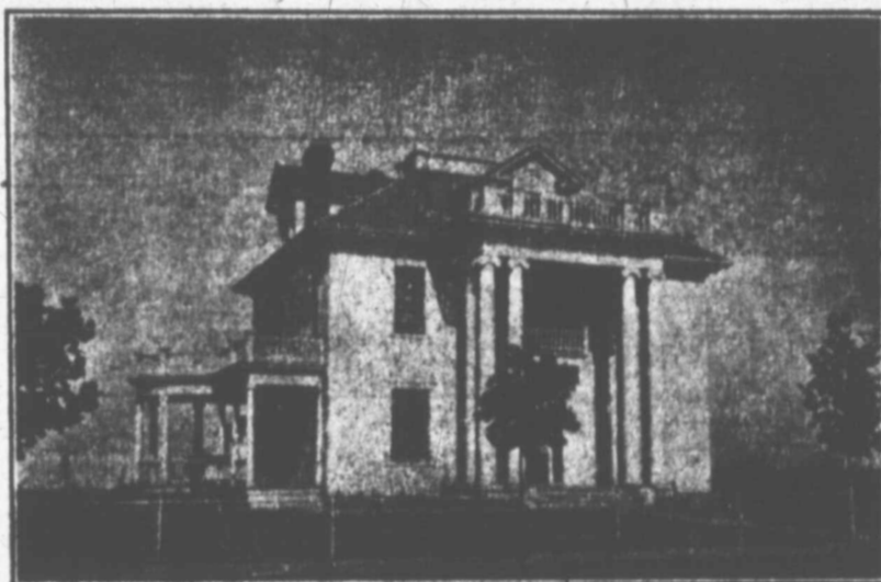
RESIDENCE OF J. L. JACKSON, DENVER AVENUE.
