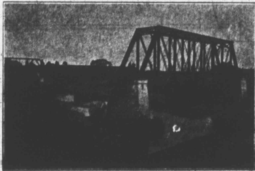
F. W. & D. C. RAILROAD BRIDGE OVER THE WICHITA RIVER.
