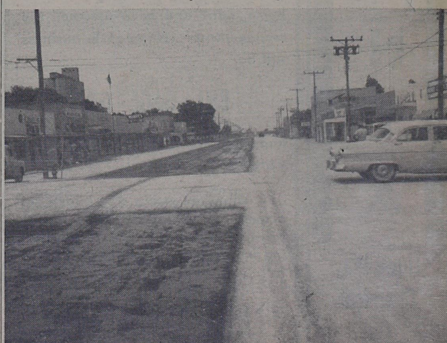
A LOT OF CHANGE — Two short weeks ago, the first strips of oil were being sprayed on Bovina streets, and now the job is finished, with the exception of additional paving under consideration on Third Street and Highway 86. Paving is one of the many improvements that came to Bovina during the past few months.
