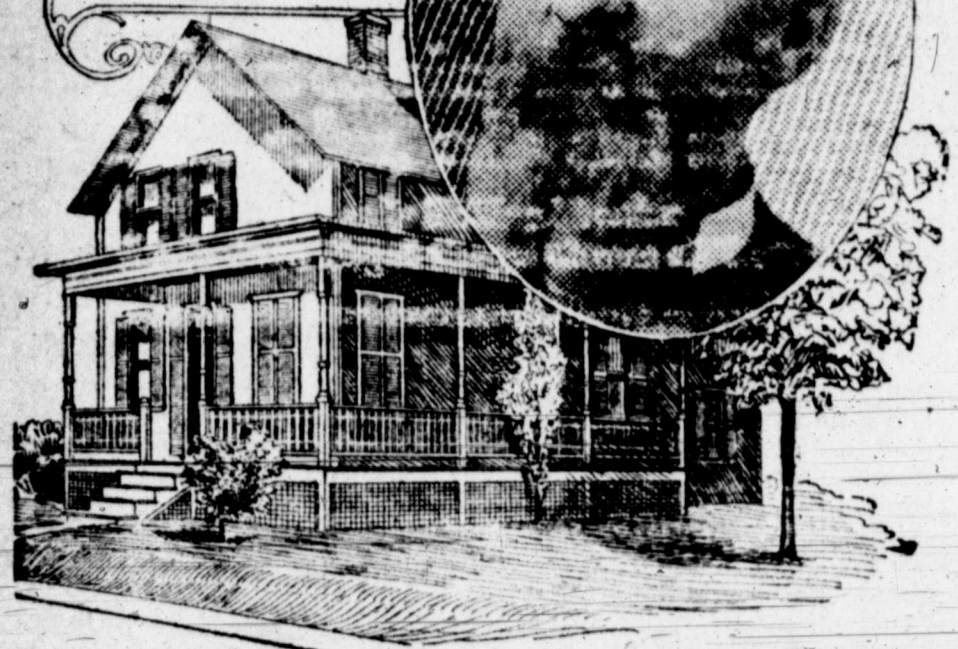
The Home of Captain Hutchinson, of Montpelier, Vt.
