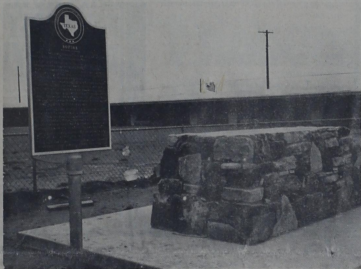
PERMANENT HOME -- Erection of the Texas historical marker at the site of the future location of the Bovina Bull was completed last week on Highway 60. The marker, presented in August at Bull Town Days, tells readers Bovina was one of the largest cattle shipping points in the nation at the turn of the century. It was placed in a permanent location before the platform, on which the bull statue, now being sculptured, will stand. The entire project is expected to be completed by 1969's BTD.
