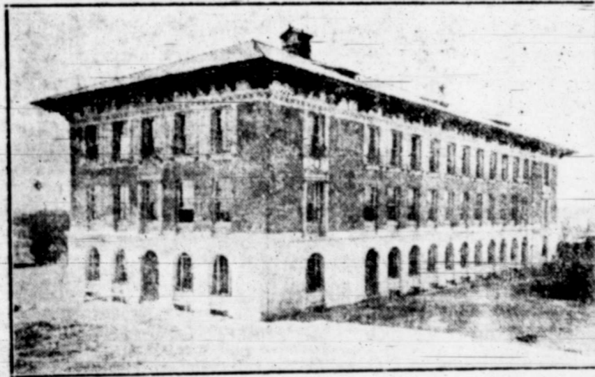
NEW EDUCATIONAL BUILDING UNIVERSITY OF TEXAS
