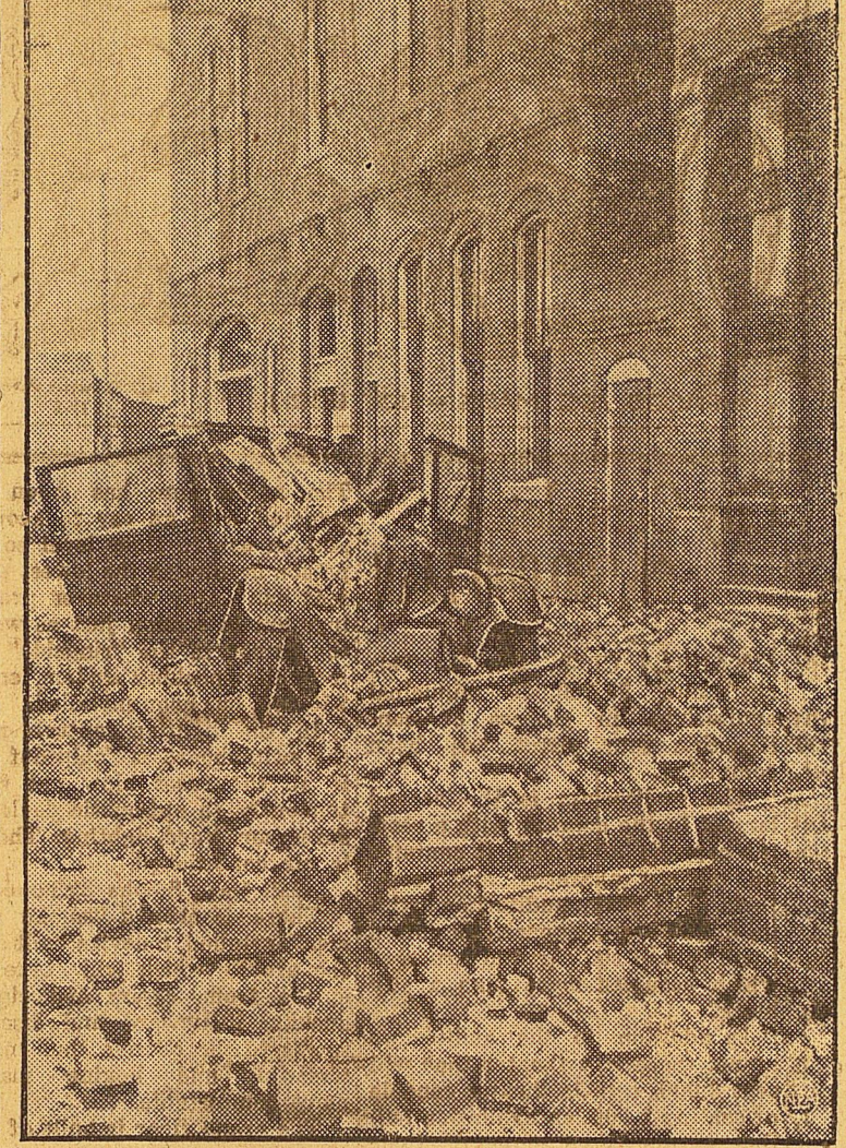
Size of the reconstruction task facing Helena is indicated by this picture, a scene of ruin along one of the capital's main streets, damaged heavily by the recurrent quakes. An automobile parked near the stores is seen after an avalanche of bricks had plunged down on it from business structures in the latest series of shocks that made thousands flee the city.
