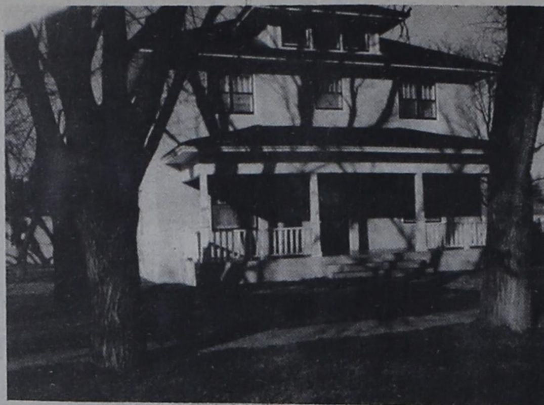
The Hopping-Aldridge House
