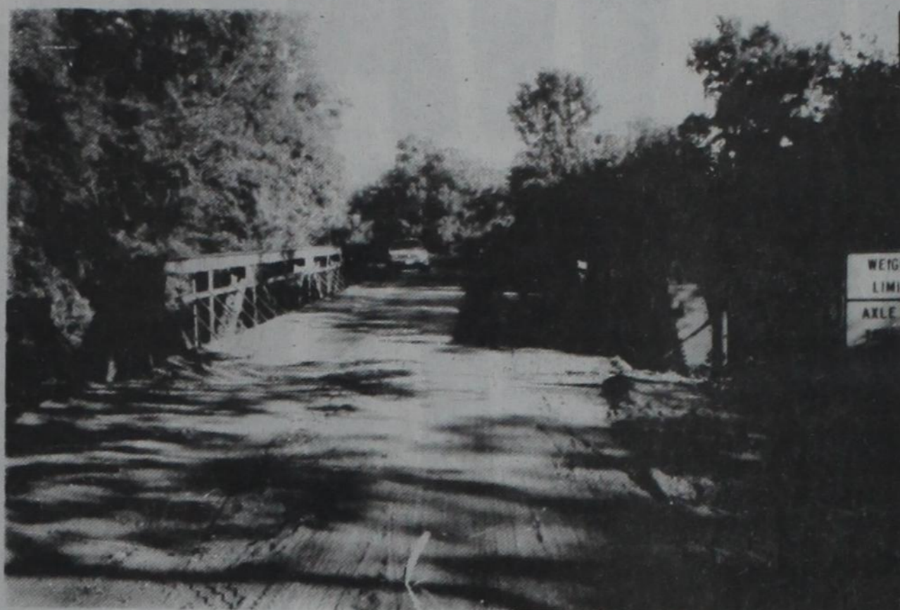
Goodbye to an old bridge. This bridge on CR 190 in Pct. 1 is being replaced by a new structure. The project will probably take around four months to complete.
