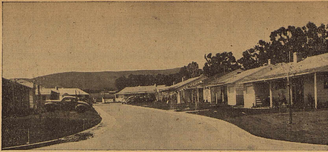
A very satisfactory type of curb and gutter has been installed in this California subdivision. At street corners the curb is vertical but along the interior lots it is sloping. This feature permits driveways to be located anywhere without cutting curbs or making special aprons. Federal Housing Administration land planning officials describe this as a practical treatment which could be copied in many low-cost subdivisions.
