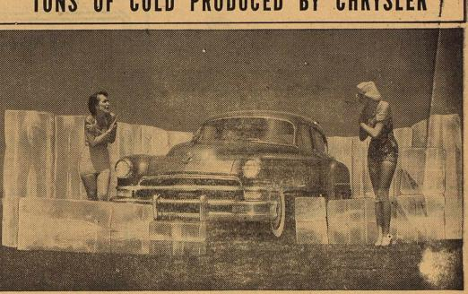
The air conditioner in this Chrysler produces cold equivalent to melting the three tons of ice shown. When a car is a broiling 110 degrees inside, Chrysler's fast cool-down fresh-air system brings the temperature to the low 70's in four blocks. The unit, which is available in Chrysler New Yorker, New Yorker DeLuxe, and Imperial models, is the highest capacity system now in use.
