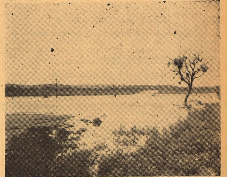
Nine Mile Crossing on the Del Rio Highway was under about seven feet of water, halting and rerouting traffic on Highway 277. The flood gauge (black dot in center) indicates depth of the flood waters at the crossing. Photo by Lovelace.
