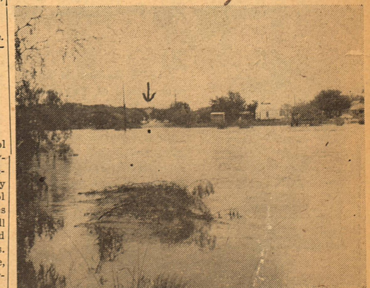
Looking across Dry Devil's River toward the Sutton County courthouse, it is easy to visualize earlier scenes described by long time residents when water backed up under the trees on the courthouse lawn. Rains of slightly greater amounts could inundate the entire business section. Photo by Lovelace.
