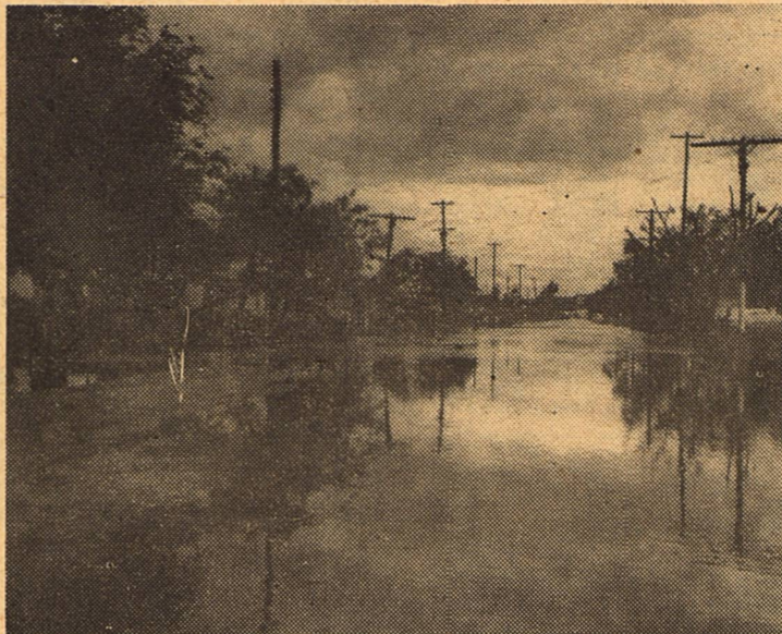
This situation which occurred during the May 12 high water on the old McKavitt road has been somewhat alleviated by the City's purchase of a lot from Wm. Cameron Co. and the excavation of a canal which will drain off excessive water. photo by Lovelace.
