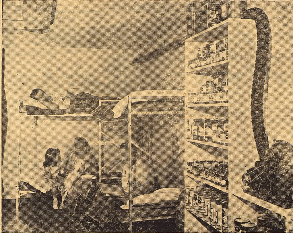
FALLOUT SHELTERS are the best way for rural Americans to protect themselves from a massive nuclear attack which could unleash dangerous radioactive fallout throughout the country. Some of the shelters recommended by the Office of Civil and Defense Mobilization are not as elaborate as this one, which includes an auxiliary generator and an electric air filtering and ventilating system. However, all recommended shelters should include the basic features shown here—a place to sleep; food, water and medical supplies, and at least eight inches of concrete or an equal weight of other materials for shielding the shelter against fallout. Free designs may be obtained by writing to OCDM Rural Civil Defense, Battle Creek, Mich. (OCDM Photo)
