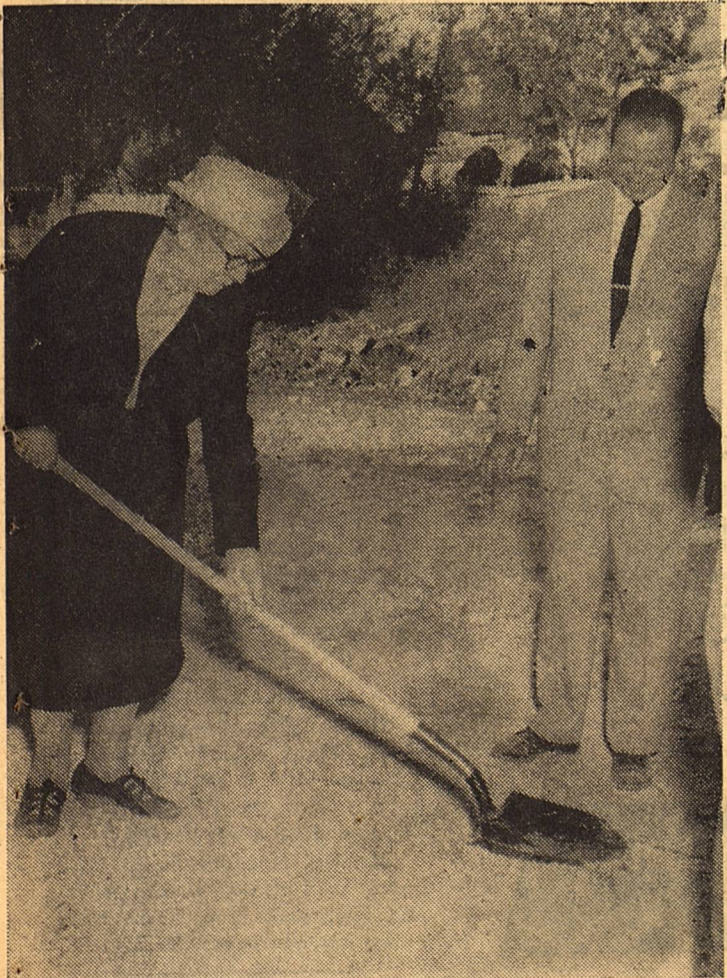
Mrs. Lee Labenske breaks ground for the building to be built soon by The Church Of The Good Shepherd (Presbyterian U. S.)
