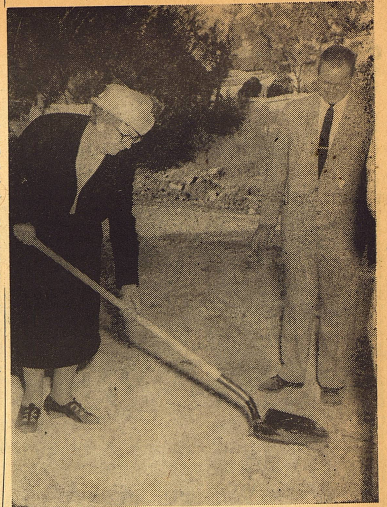
Mrs. Lee Labenske and the Rev. Allan Guthrie were among those breaking ground for the new Church of the Good Shepherd building now under construction. Ground breaking services were held in September and plans call for occupation in April 1960.
