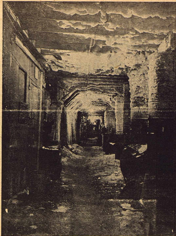
This long tunnel beneath the snow at the South Pole Amundsen-Scott station in the Antarctic connects the scientific building and the mess hall.
