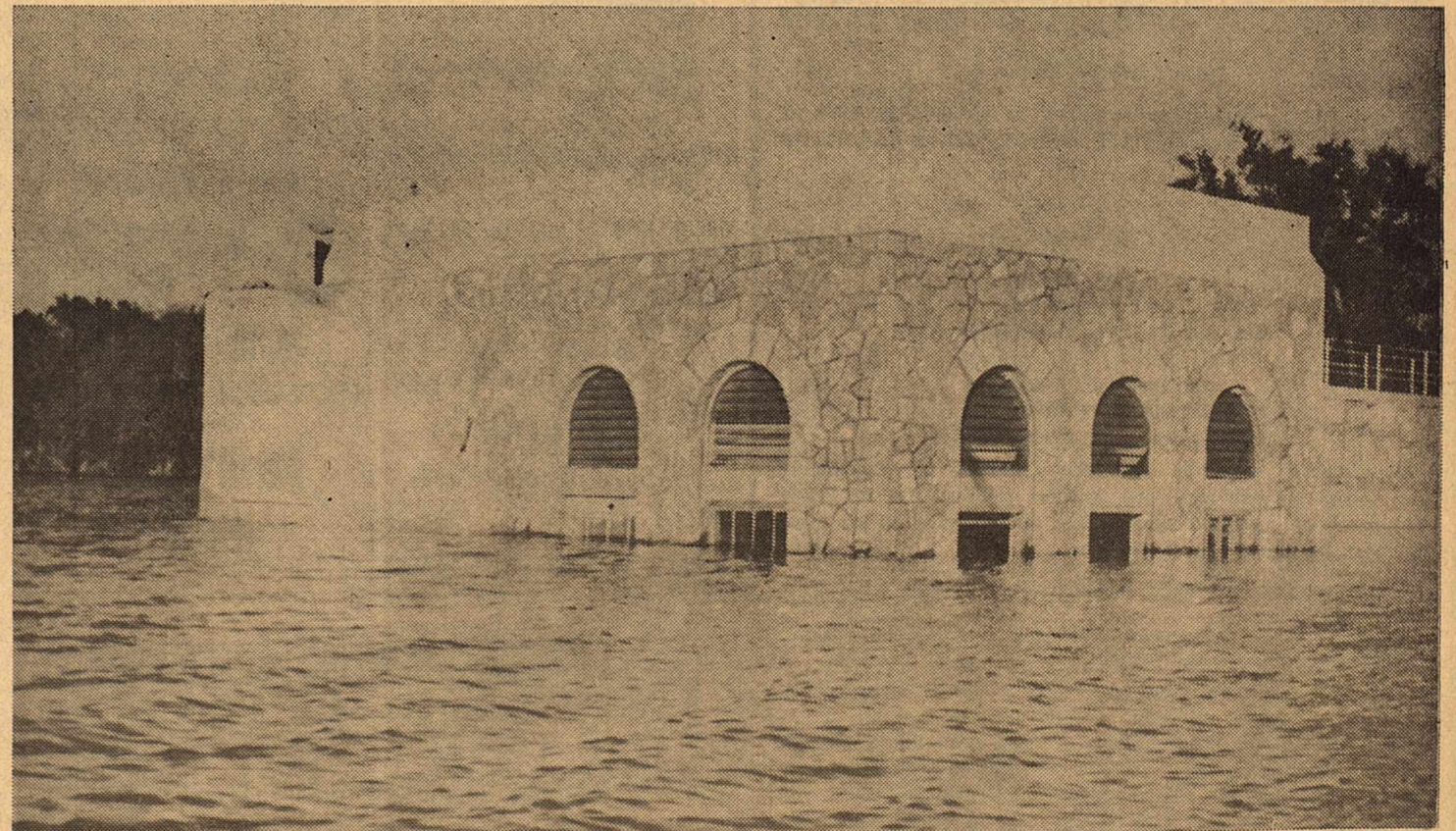
AMISTAD LAKE, which will probably eventually be the fisherman's paradise, is rapidly filling as evidenced by water level on the lake dam power house. Amistad Lake has approximately 146 feet of water now. Amistad reservoir is located in Val
