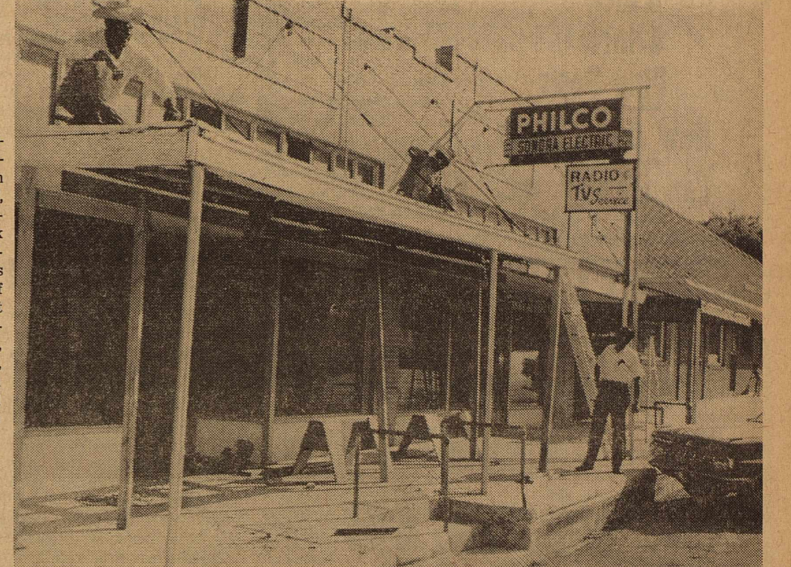
AWNING ALTERATION is taking place in front of the Elliott Building and Sonora Electric. Nelson Stubblefield, who shortened his awning over the electric company, plays sidewalk superintendent while Mike Duran and Mike Jr. work on the Elliott Building. Heavy spring rains put the final touches on rotting edges of the awning.
