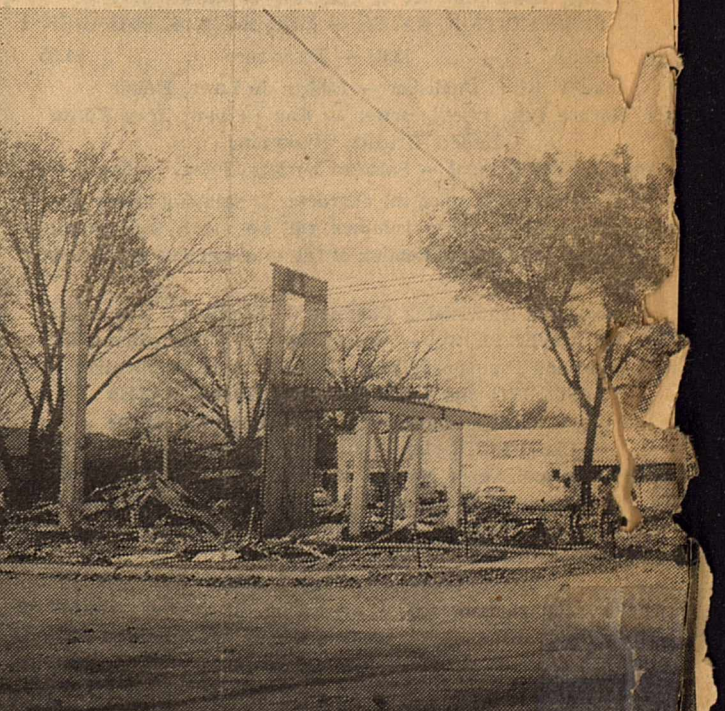
LAST ITEMS TO BE TORN DOWN were the southeast corner of the porch and the chimney. The remaining trash from building is presently being removed from the site. The remains are a reminder of the years of community life centered around the famous landmark.
