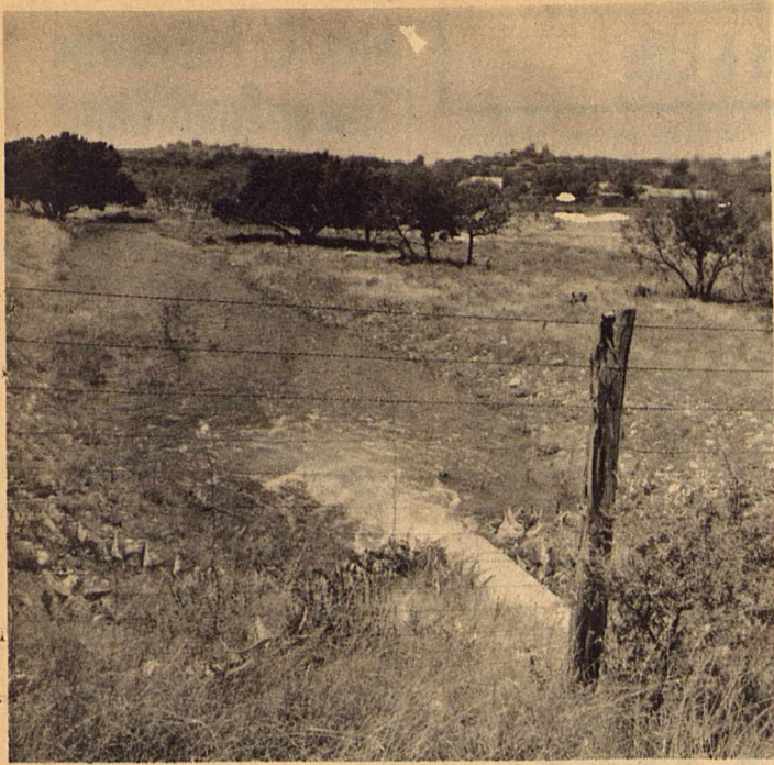
THE FLOOD WATERS from last week's rains at structure No. 13 have been slowly released through the principle spillway to prevent downstream flooding.
