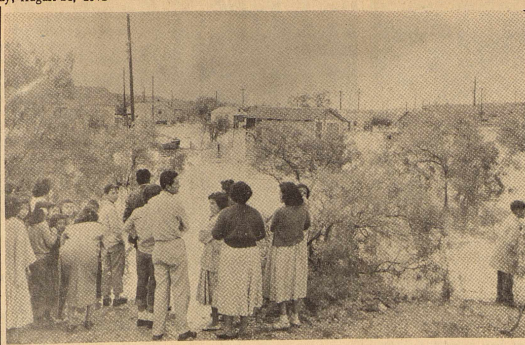
SOME RESIDENTS ANXIOUSLY watch rising flood waters of Dry Devils River and Lowrey Draw invade their homes after a 3.5 inch rain-fall May 12, 1967. The thirteen watershed dams above Sonora protected this same area
