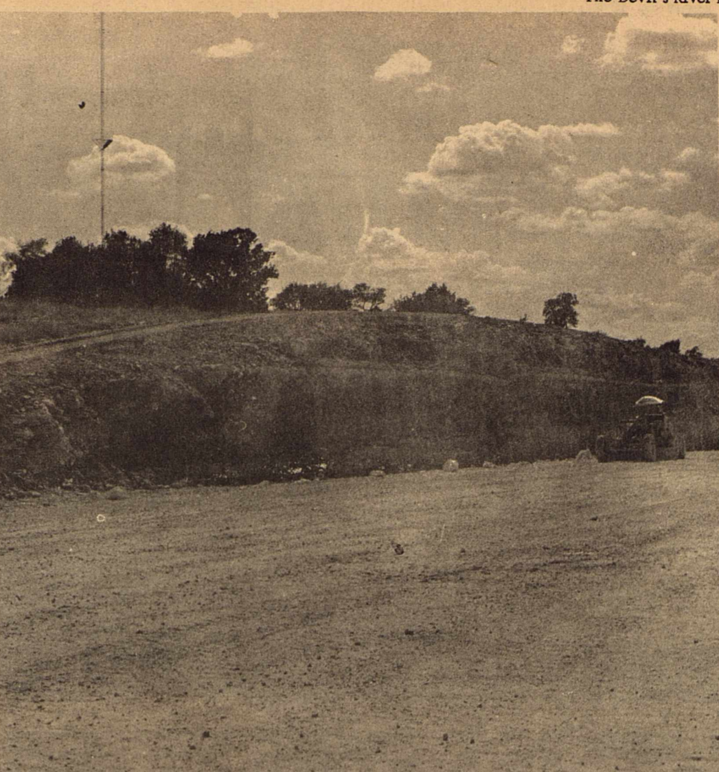
THIS AREA OF IH10 CONSTRUCTION was the scene of a freakish accident last week when Monte Dillard went over the 25-foot embankment on a motorcycle. Fortunately, his in-
