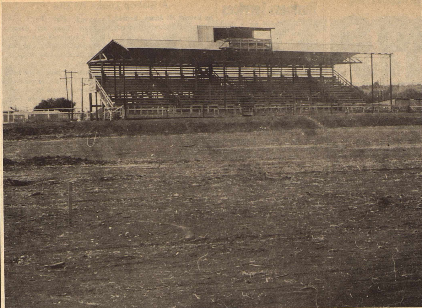
The old rodeo arena at the Sonora Park Association Fairgrounds has been cleared to make room for a larger and more modern arena. Improvements to grandstands are
