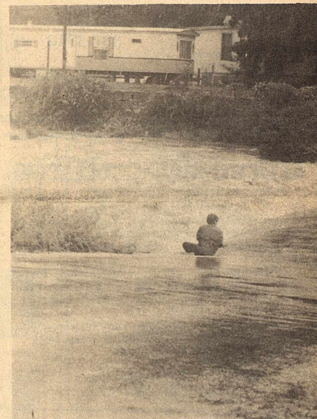
Water Street crossing (the dip) was closed for five days.
