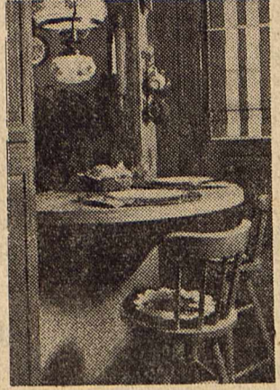
Cut-through above snack bar allows communication with guests and enjoyment of living room's picture window. Cans are stored in shallow cabinets between studs to either side of opening. Traffic moves easily around the counter. Stools slide under.
