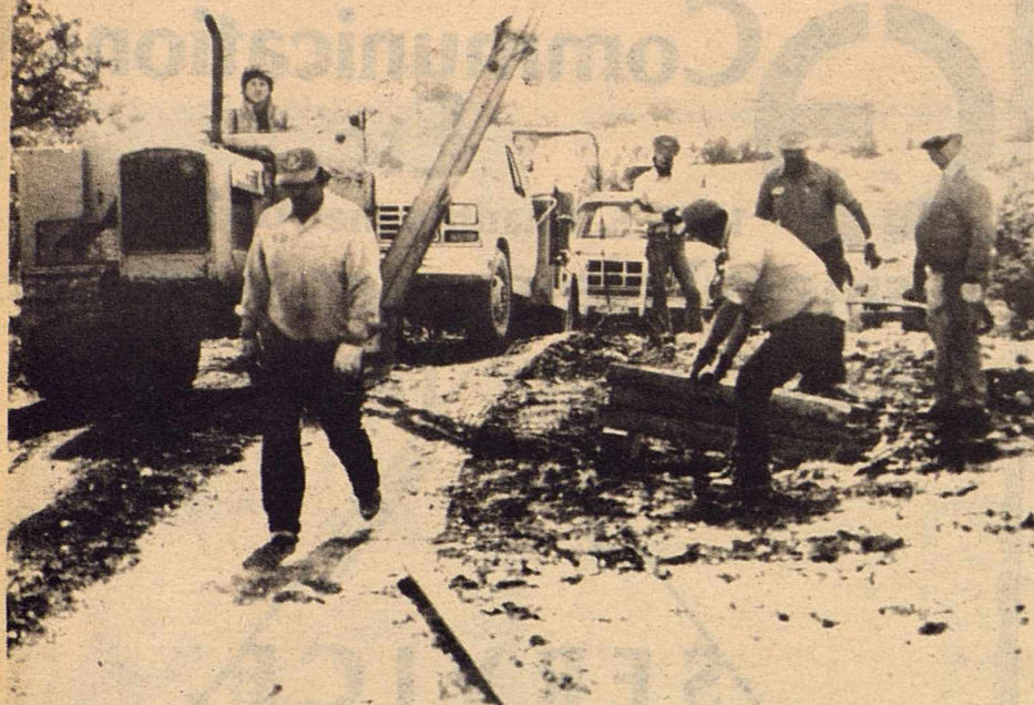
Construction readies site.
