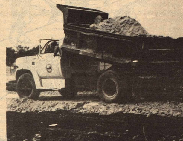
DUMP TRUCK UNLOADS SAND FOR RIG SITE.
