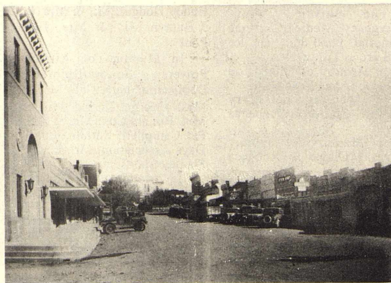
This picture of Main Street was taken shortly after the completion of the 1928 First National Bank Building.
