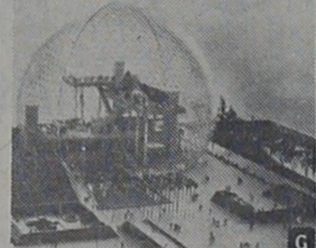
One of the attractions at Montreal's Expo 67 is the U.S. Pavilion housed in a 20-story-high geodesic dome designed by Buckminster Fuller.
