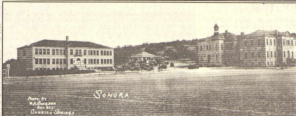
School campus after 1930 new brick high school was built
