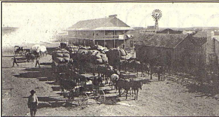
Intersection of Main and Concho Streets, Murphy home, Devil's River News, Commercial/McDonald Hotel, Livery Feed and Stable to right of hotel and Drake/Aldwell home to rear. You can also see the windmill and tank that were second waterworks in Sonora.
