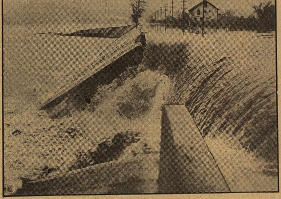
Through this huge gap ripped in Beechmont levee, Cincinnati, by the Ohio river's pounding flood waters a roaring torrent poured down on lowlands, converting them into a shallow sea and inundat-ing Lunken airport. Even on the higher land seen in the background the water rose to a threat-ening level, in the third greatest deluge in Cincinnati's history. Most of the city was high and dry, with business as usual, but transportation was seriously affected.
