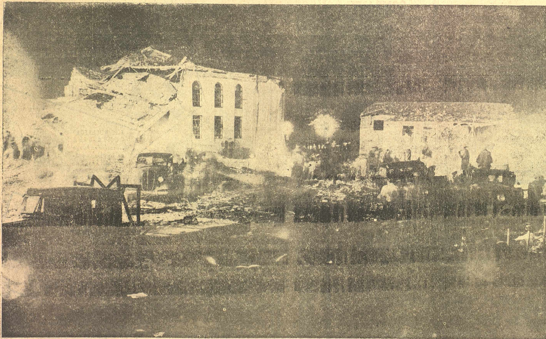
A night shot of the tragedy. At left is the school auditorium in which scores of children died. The building on the right is one wing of the school. The demolished structure formed an E in the foreground of the picture, connecting with the wings which remain. This unusual picture as he stood on one of the oil field trucks which were used to pull the wreckage apart in the search for bodies.
