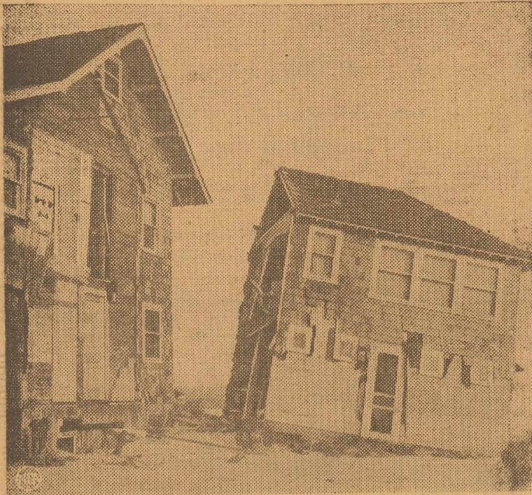
Cut cleanly in two by the hurricane but still standing, this house at fashionable West Hampton, Long Island, was one of the many freaks of the storm that laid waste great areas of the eastern seaboard. A wing was torn from the main section of the house.
