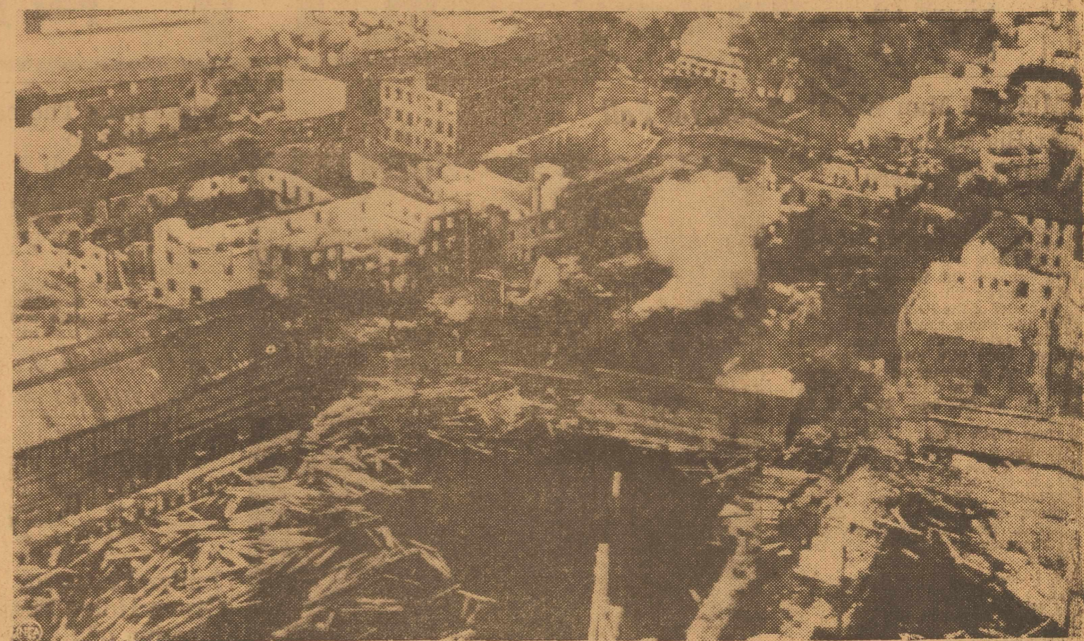
This air view of New London, Conn., showing buildings unroofed and wreckage strewn everywhere tells a graphic story of the havoc wrought in the New England states. Fire followed flood and blazing ruins can be seen at the right, center. Note the backwash of lumber in the shipways in foreground. With the death toll mounting hourly, the number of missing was a matter of guesswork. New London is a historic New England whaling center.
