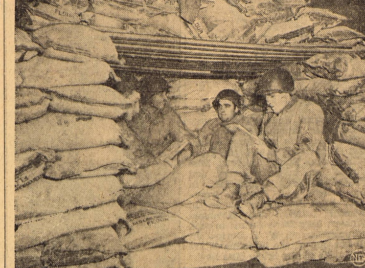
Ingenious Yank soldiers attached to a G. I. bakery near Anzio beachhead targets often bombed and strafed by Germans contrived the snug air-radiated shelter pictured above—out of flour bags instead of sandbags. The mobile bakery turns out 13,000 loaves of bread a day.
