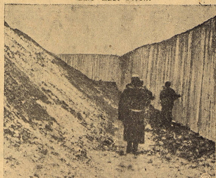
The photo above, just received from neutral sources, shows Nazi soldiers walking along bed of 20-foot deep anti-tank ditch, buttressed by wall of reinforced concrete, said by Germans to be part of Hitler's "Atlantic Wall" defenses against Allied invasion.
