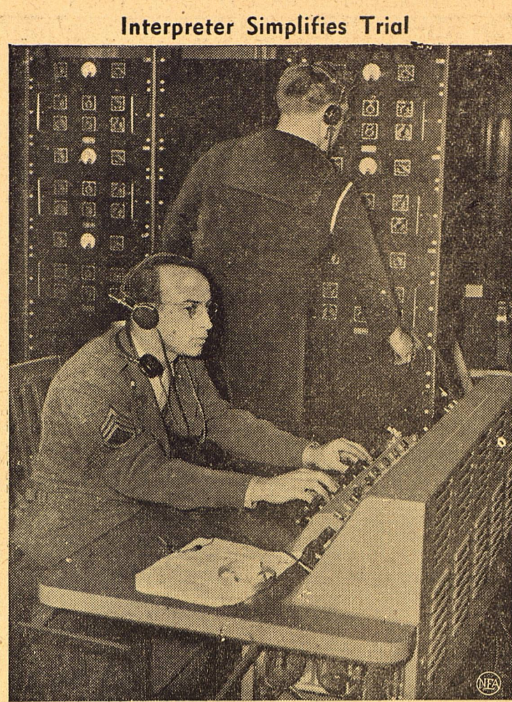
Through the use of this novel electrical system, Nazi defendants in the Nuernberg war crimes trials are able to hear instantaneous interpretations of procedure and evidence in any one of four languages. Army and Navy technicians operate the control boards.
