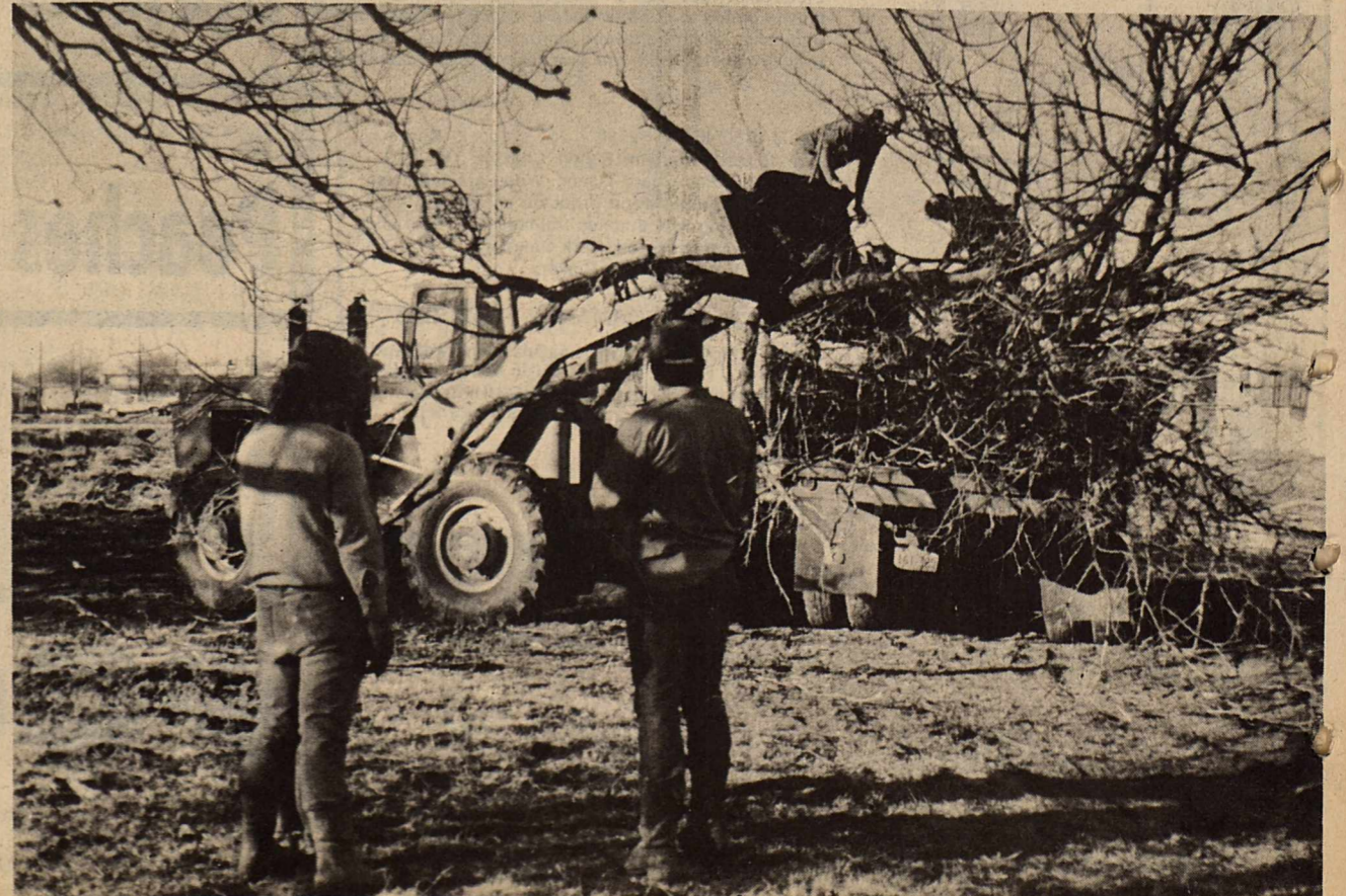
DONATED EQUIPMENT REMOVES DEBRIS
