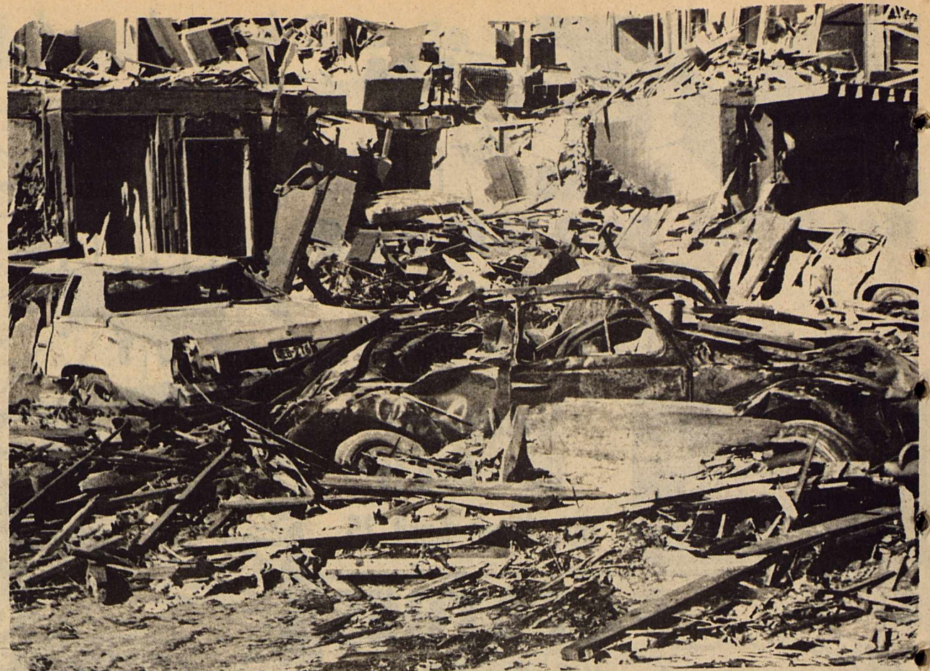
RUINS OF APARTMENTS and autos in Wichita Falls... Representatives from the towns of Wichita Falls and Vernon have stated that they no longer need clothing and other similar goods for storm victims as donations
