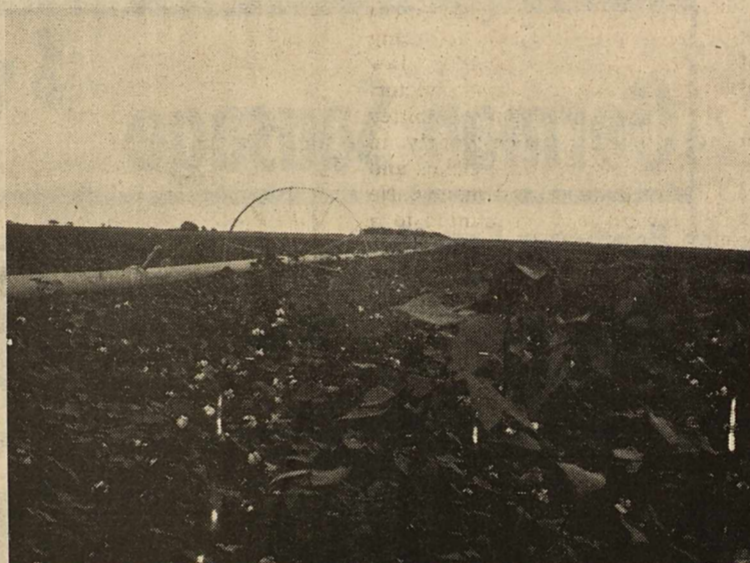
14,908 feet of irrigation pipelines were installed for water and energy conservation.
