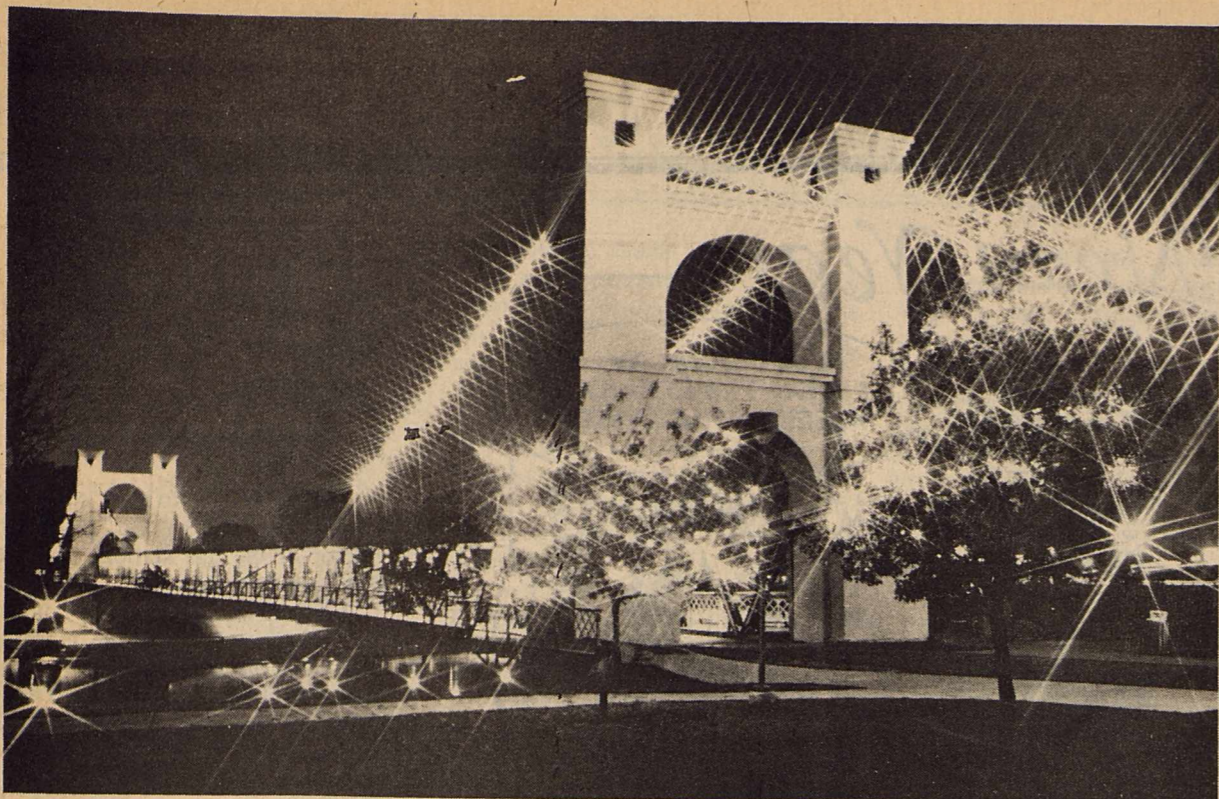
The Waco Suspension Bridge was the longest of its kind in the nation when it was built back in 1870. Thousands of cattle and numerous wagon trains passed over the structure in its heyday, and the famous Brooklyn Bridge in New York was patterned after it. The 475 ft. bridge is still used today, but only as a pedestrian crossing. Tourism Division, Texas Dept of Commerce photo.
