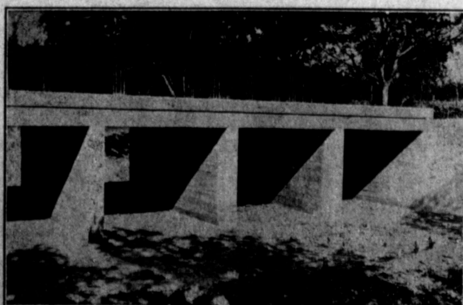
CONCRETE BRIDGE OVER DRY BRANCH, ON THE NEW HIGHWAY
