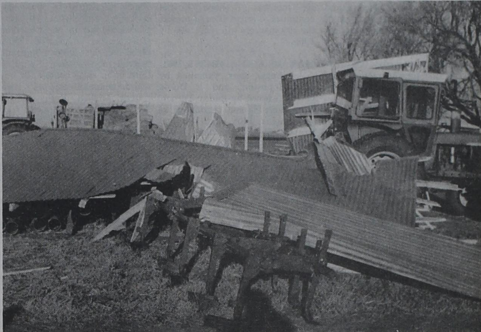
HIGH WINDS....High winds Monday night caused considerable damage in the area. Pictured above is a 60 foot roof of a hay barn on the McCain farm that blew off and broke a window of a tractor several yards from the barn. Winds were clocked at over 50 miles per hour.
