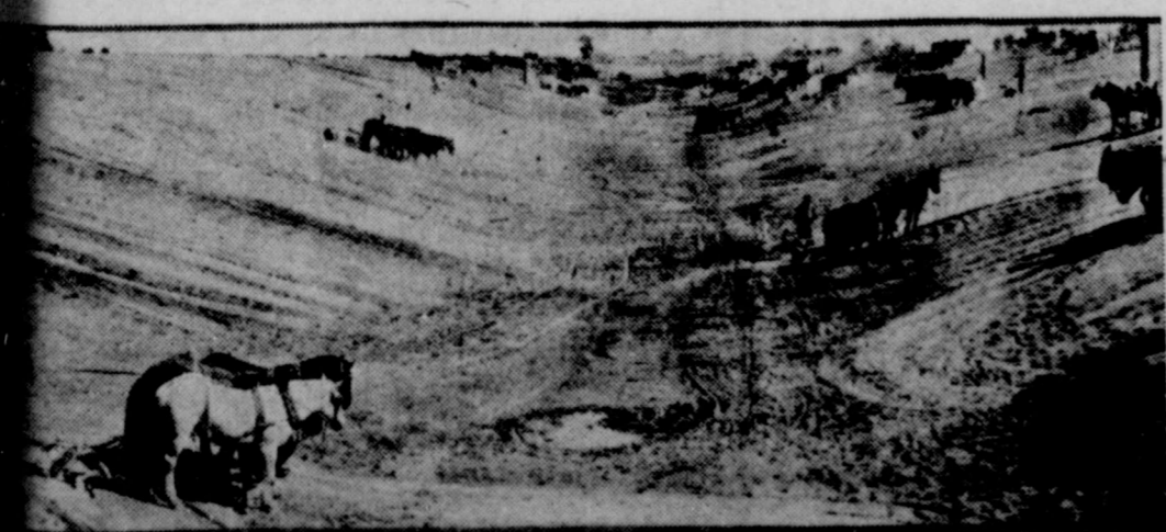
Hundred four-horse teams are here busy on one section of the All-American canal which will replace the old Colorado river 80 miles across the valley for irrigation purposes. The new canal will have a width of 232 feet, a depth of 10 feet and will carry the water of the Colorado river 80 miles across the valley for irrigation purposes. The teams shown in the photograph above have moved more than 1,000,000 yards of earth with their trappers.
