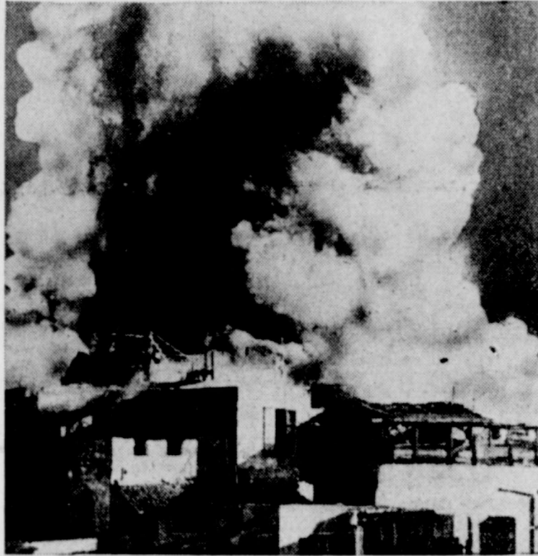
This unusual picture shows houses in Jaffa, Palestine, being blown into the air by the force of an explosion. In one week 150 houses in the old city were blown up by British troops as part of their plan for the defense of Palestine. Steel helmeted troops armed with machine guns surrounded the old city during the operation.
