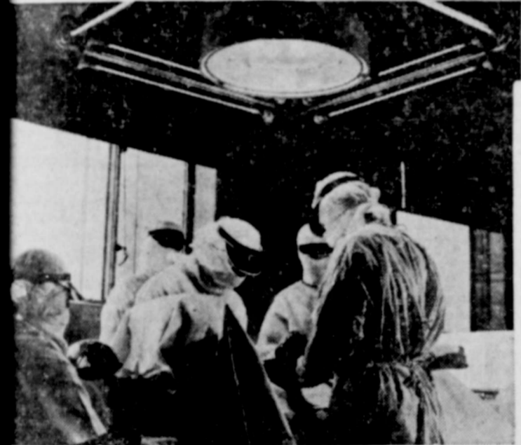
How ultraviolet radiation purifies the air in an operating room, eliminating danger of infection from bacteria in the atmosphere. Note "sterilamp" in the ceiling, the long tube-like lights.
